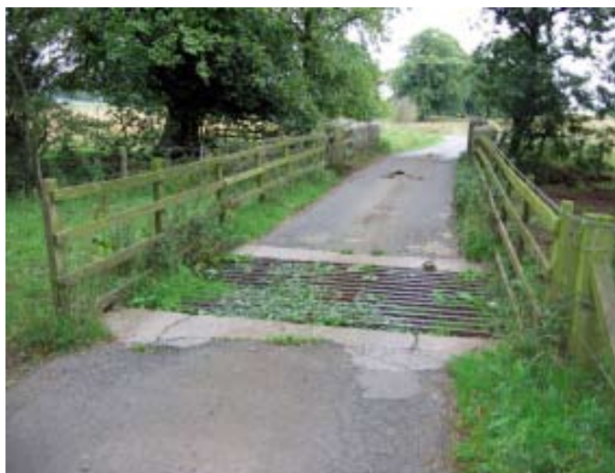
Below: Fenwick, Northumberland. Riders are forced to turn at ninety degrees through a small gate, and go well outside the bridleway. Illegal and unsatisfactory.
